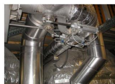
3-way valve for segregation of effluents
