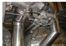
3-way valve for segregation of effluents
