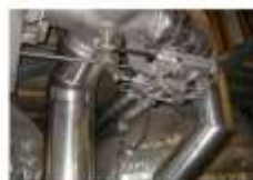
2-way valve for segregation of effluents
